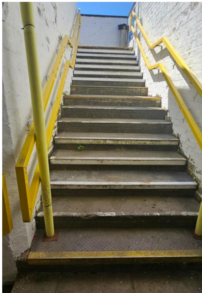
Fig.10: Stairs leading up to Platform 2 (cont.)
