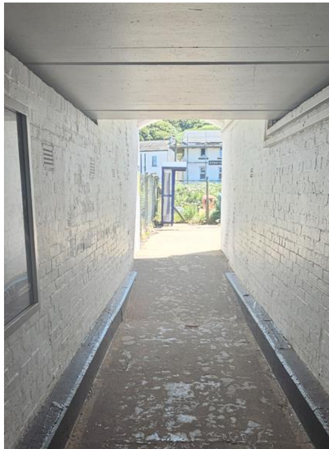
Fig.8: Underpass entrance incorporating a gently sloped access ramp at the approach.
