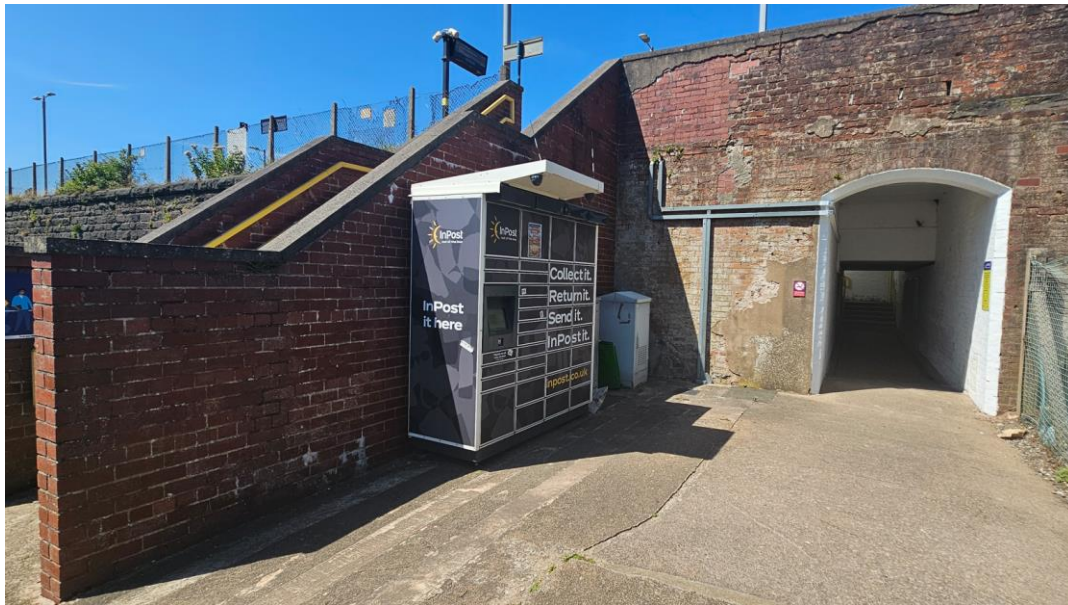
Fig. 5: Stairs providing access to Platform 1 are located to the left, with an InPost machine and electrical cabinets positioned along the stair wall. The underpass entrance is located to the right.
