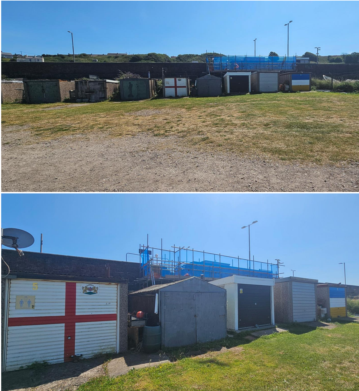
Fig. 11&12: Garages behind Platform 2.
